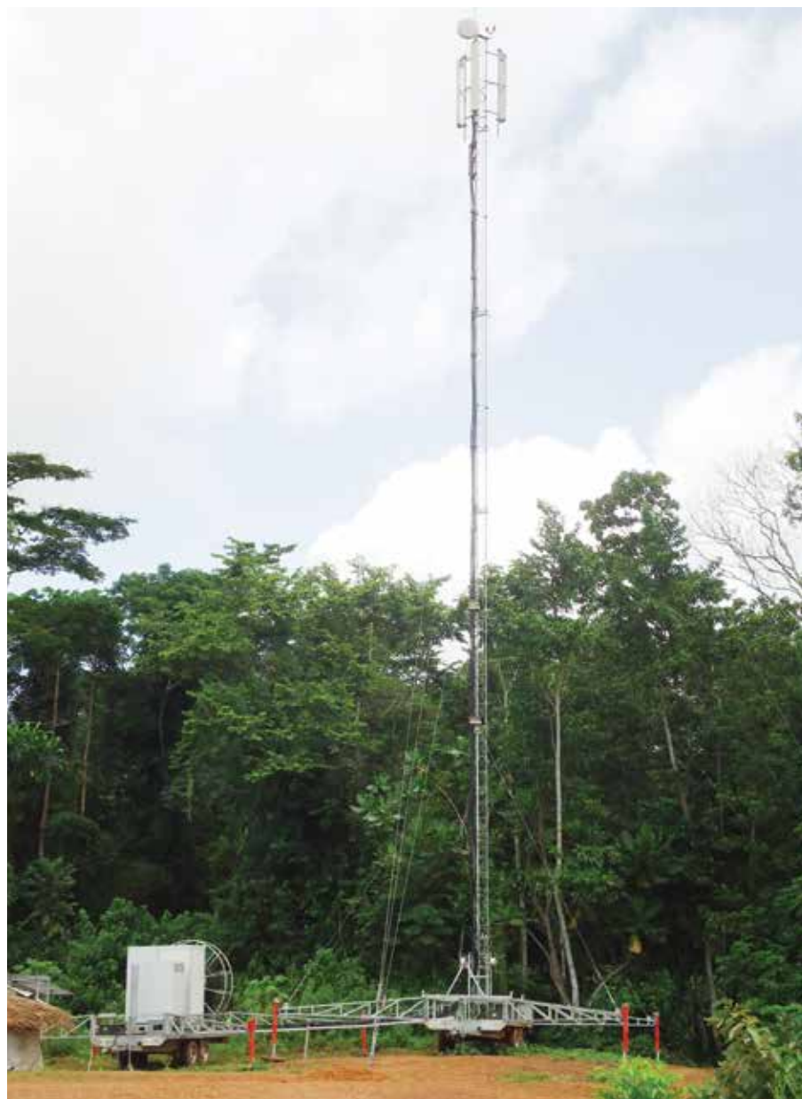
A new mobile tower gets erected at the camp
