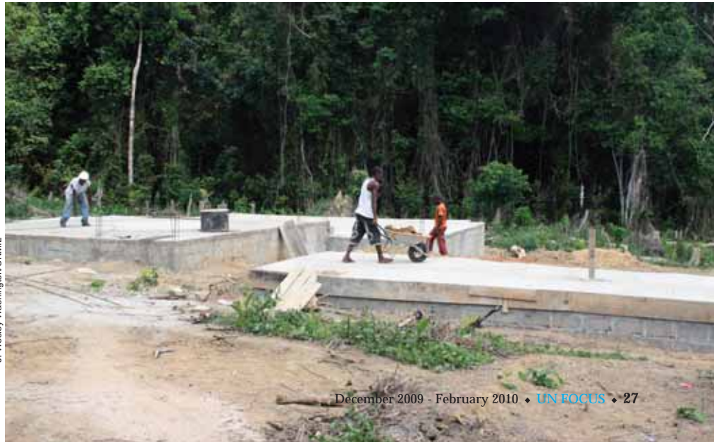
A primary health clinic under construction in Rock Crusher, Kokoya District
